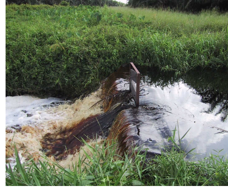
Control structure in oil palm plantation in Central Sarawak to maintain high water levels.
