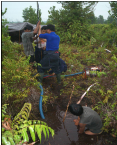
11. Drilling deepwell and stay in the tend
